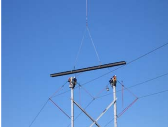
Picture 2. Live (energized) installation of FRP Cross Arm with Helicopter Lift
