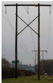
Picture 1. Timber/Wood H-Frame
