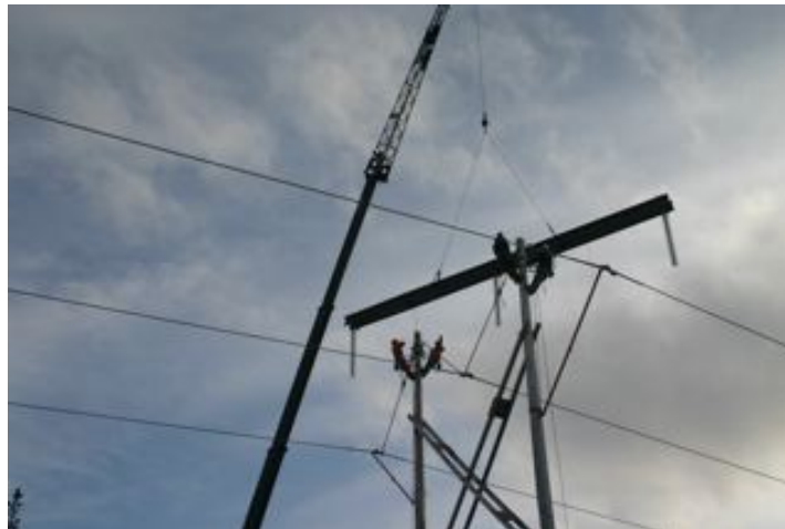
Picture 3. Live (energized) installation of FRP Cross Arm with Crane Lift
